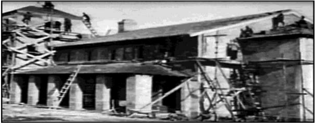
The ensemble of the Albanian-American Institute of Kavaja (Near East Foundation) The Boys' Building during construction in 1930, under Meyer's supervision. ( Cafeteria and Theatre Building )
